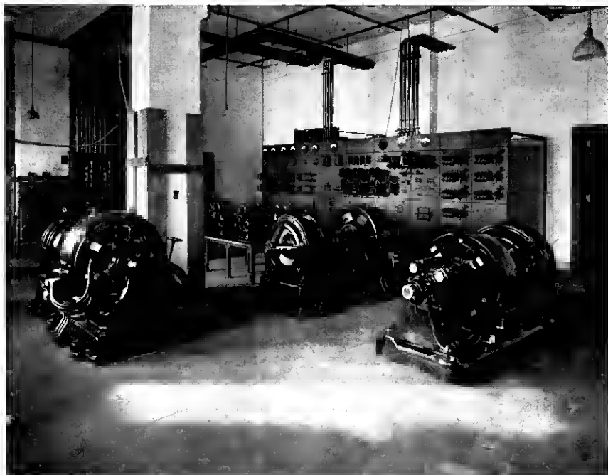
Fig. 15—Power Machine and Control Equipment for Two 10,000-Line Units
