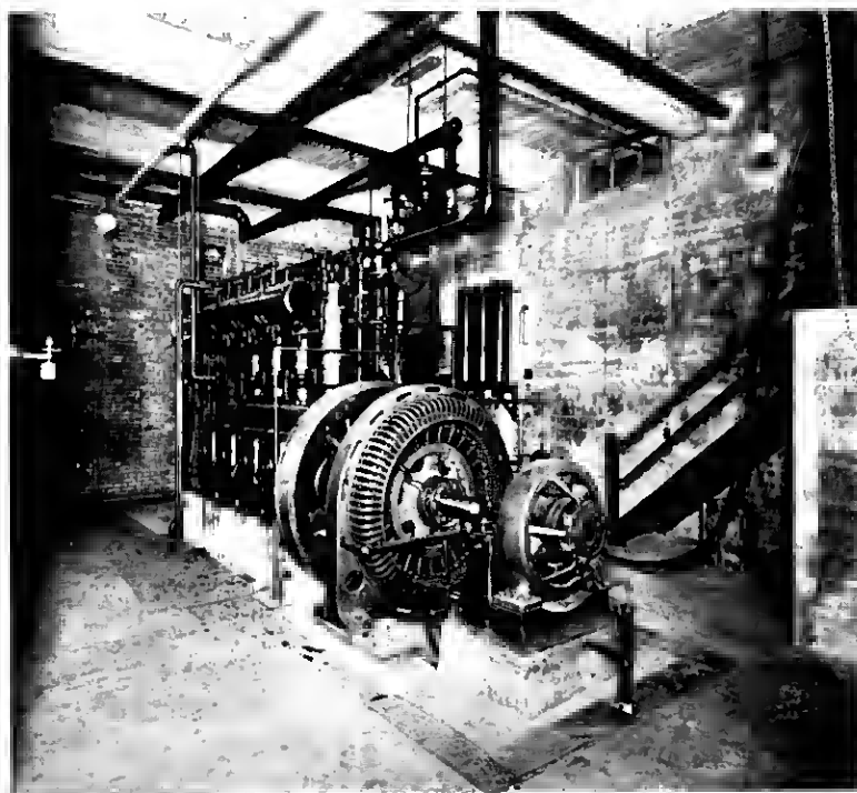
Fig. 17—165 H. P. Gas Engine Generating Set for Emergency Use
