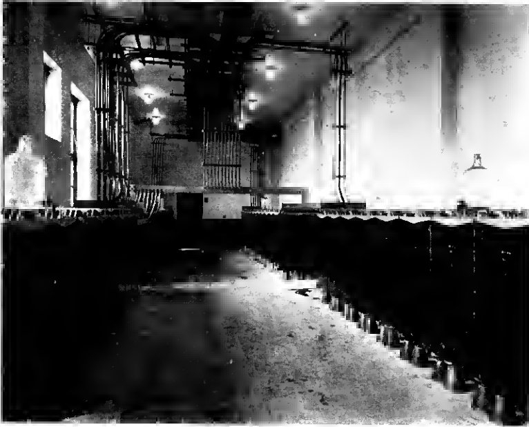
Fig. 16—Battery Room for Two 10,000-Line Units
